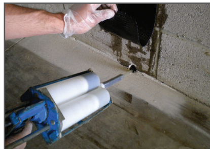
Apply epoxy to hole
