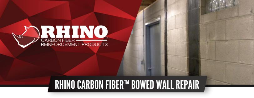
When foundation walls start bowing or moving inward, it is a sign of structural failure which should be addressed immediately. The primary causes for bowing walls are: outside hydrostatic pressure on the walls from soil, tree roots and construction failures/poor quality construction (ex. improper steel reinforcement resulting in excessive load due to ineffective tensile strength transfer to the wall).
